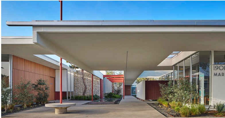
Main Entry to Mariners Medical Arts Building Credit: Benny Chan/Fotoworks
