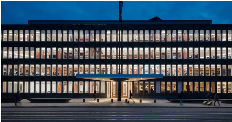
View of the restored main façade of the former U.S. Embassy in Norway, which now has recovered the original black color of the precast concrete Credit: Einer Aslaksen
