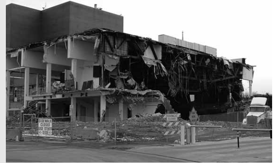
Demolition of Guthrie Theater, Minneapolis, MN, 2006 (photo: Mike Rogers, manyhighways.com)
