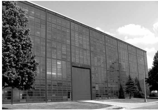
Exterior, Building 521, Great Lakes Naval Station, IL (photo: Cody Wright)
