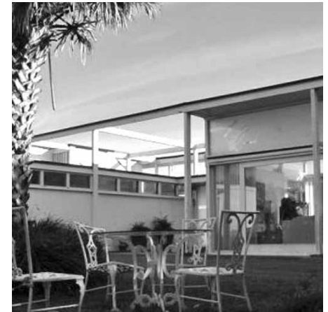
Front Perspective with detail of clerestory windows (photo: Andrew Roman)
