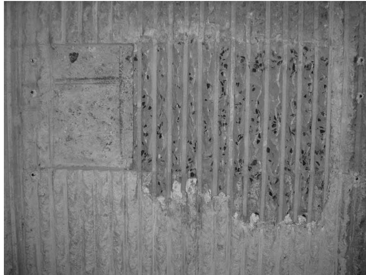
Testing the making of the vertical 'corduroy' ribs and the adhesion of new concrete to the old, Art & Architecture Building, detail, New Haven, CT. (photo: Hilary Sample)
