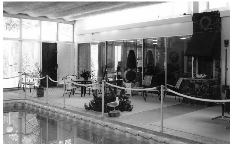
Natatorium, with steel paneled ceiling
