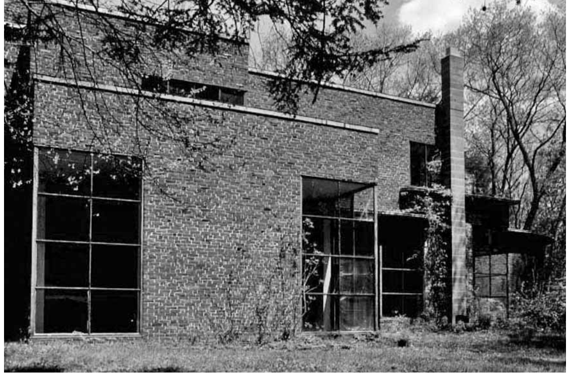
Rear façade, Wells House, Southbridge, MA, 1933 (photo: David Fixler)
