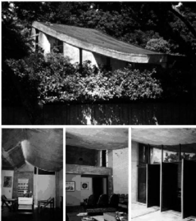
Figure 2: Paulo Meirelles Residence, project by Marcos Domingues da Silva, 1968. 1. Exterior; 2. Shed (skylight); 3. Interior with air brick panel (cobogó, hollowed out element pre-molded in plaster cement); 4. Pivoted doors with Venetian blinds.
