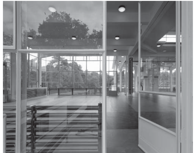
Carefully reconstructed parts such as the steel window casements, the sheet glass and the linoleum floorings. (Photo: Jannes Linders)
