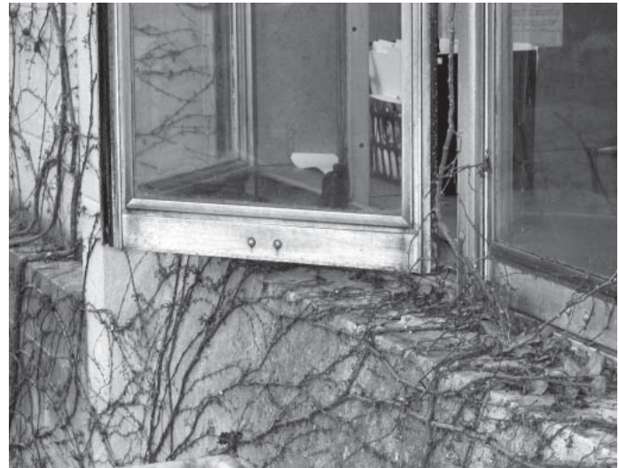
The unusual bi-fold windows at the Administration Building require frequent repairs. Parts are no longer available
