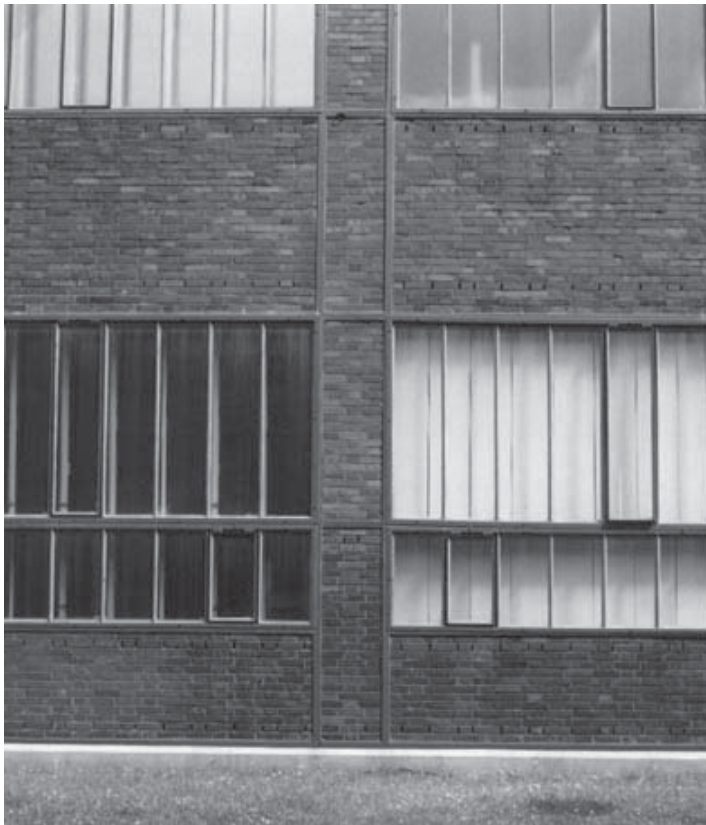
Detail of renovated curtain wall.
