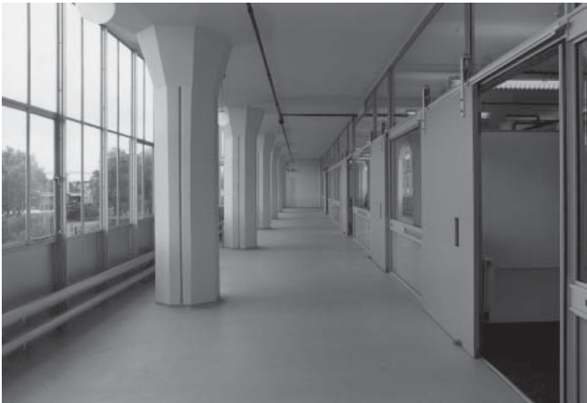
At the shadow-side, the secondary glazing is located at some distance from the original facade leaving enough space for corridors. At the other side, the sun side, the glazing has been placed between the columns, corresponding with the position of the original sunshades, creating a climate-regulating wall. (Photo: Fas Keuzenkamp)
