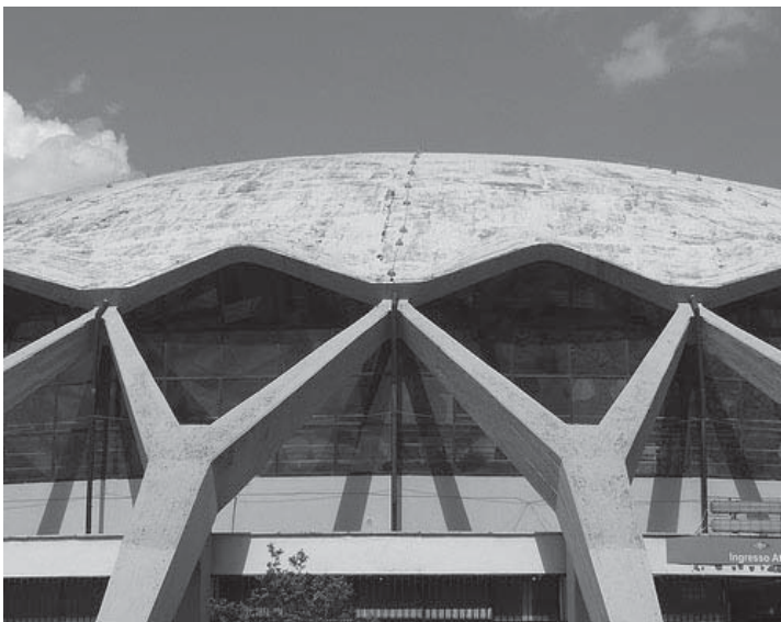
View of Nervi's concrete Y-shaped trestles, Sport Palace, Rome. (Photo: Sarah Rinehart)
