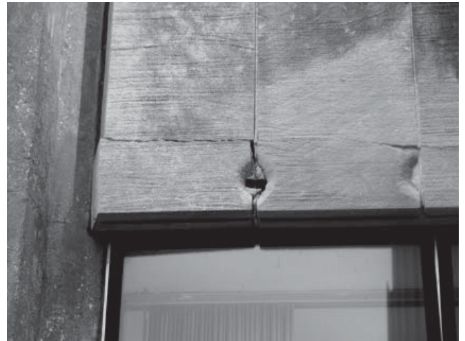
The thin stone panels on the Laird Bell Law Quadrangle are deteriorated due to corrosion of the steel anchors.
