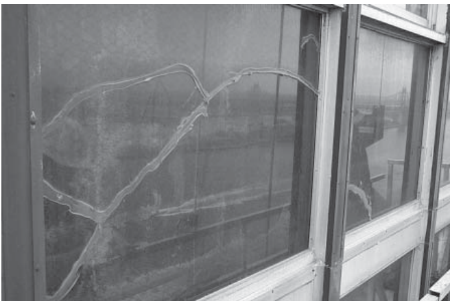
Cracked and sealed spandrel glass.
