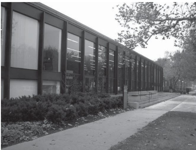
The School of Social Service Administration (Ludwif Mies van der Rohe, 1965) has experienced glass breakage from corrosion of steel elements.
