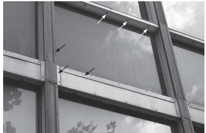
Remedial aluminum covers and weep hole plugs, c. 1952.
