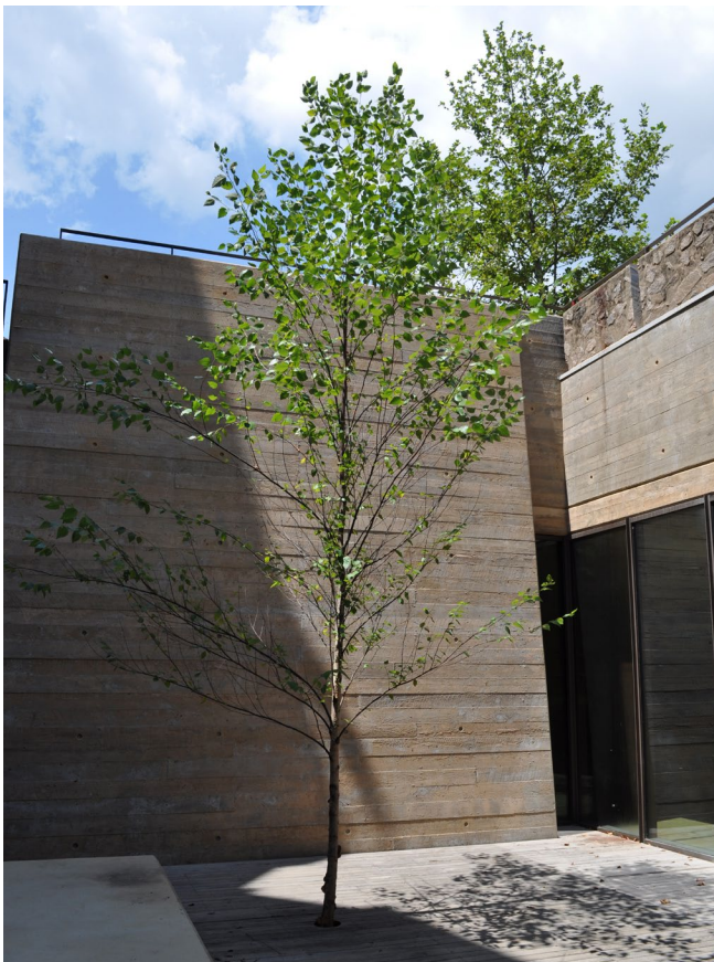
Board formed concrete walls, slightly battered, that were part of the addition. The original construction also included board form concrete walls.
