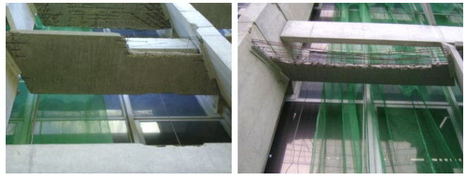
FIGURE 5: CELPE building, brises with high degrees of deterioration (to be replaced). Source: CONCREPOXI, 2009.
