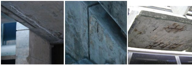
FIGURE 3: CELPE building slab canopy damage (efflorescence), detachment of the concrete, brise corroded with concrete detachment. Photos: Barbara Aguiar (left, center) Source: CONCREPOXI, 2009 (right)
