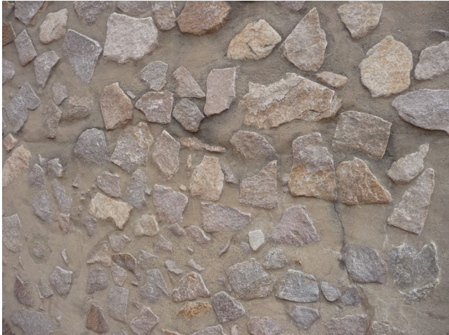
Close-up of rubble concrete, showing a crack on the right side and various levels of soiling.
