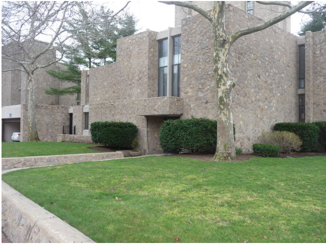
Overall view of rubble concrete walls with inset windows.
