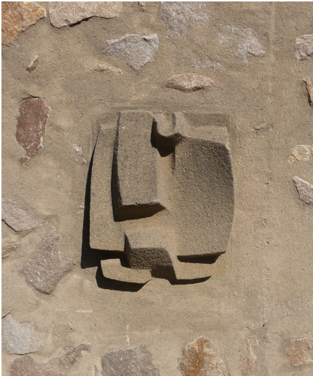
Concrete sculpture with smooth finish embedded into rubble concrete wall. The sculpture appears to have been mortared in place after construction of the rubble wall.
