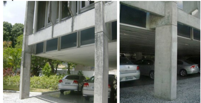
FIGURE 7: CELPE building, south facade in 2008 before the intervention. Pillar presenting moisture stains and corrosion and the same location in 2012. Pillar recovered in 2009 without major visual differences to the original structure. Photo: Concrepoxi (2008) (left) Fernanda Herbster (2012) (right)
