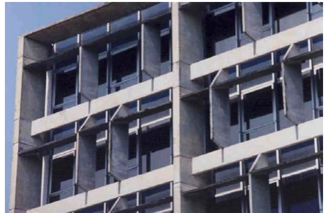
FIGURE 2: CELPE Buildings, Detail of the front façade detail of CELPE with vertical and horizontal brises. Photo: Ana Holanda (2011).
