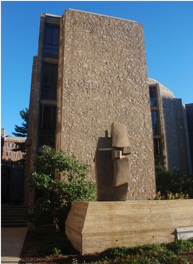
Rubble concrete wall with board form concrete in the foreground. Also note the decorative sculpture.
