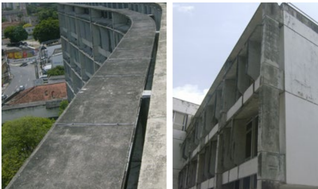
FIGURE 4: CELPE building, Stains caused by acid soot and moisture, generalized spots. Source: CONCREPOXI, 2009.
