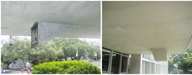
FIGURE 8: CELPE Building, main entrance slab in 2008, before the intervention, with its original rusticity of exposed concrete, and in 2012, free from deteriorative processes, but coated with paint, including the gargoyle Photo: Ana Holanda (2008) and Fernanda Herbster (2012).
