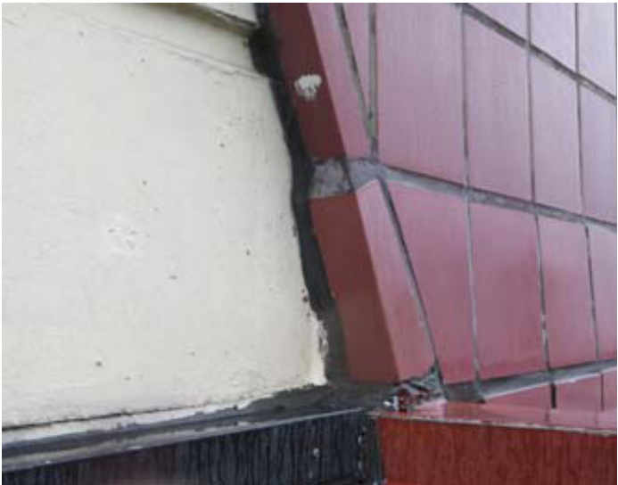
Modified tiles at keystone with irregular joints/alignment
