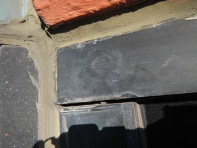
Complex material transition joints dependent on sealant
