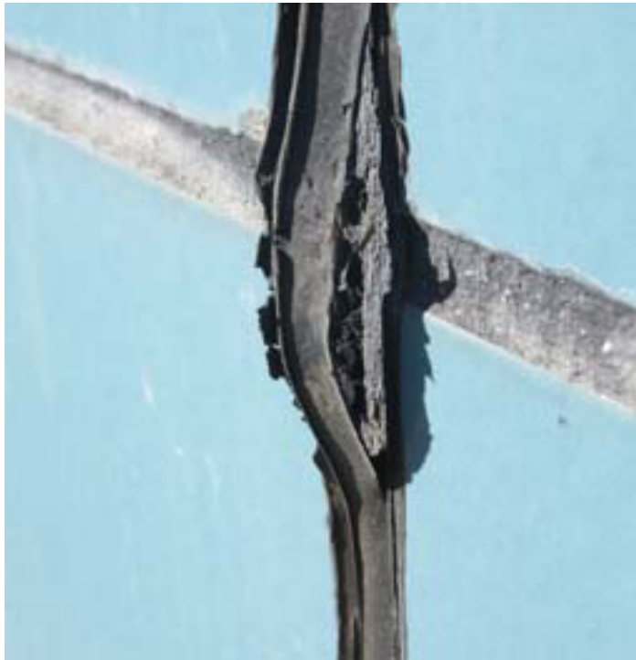
Failed sealant at tile system control joint
