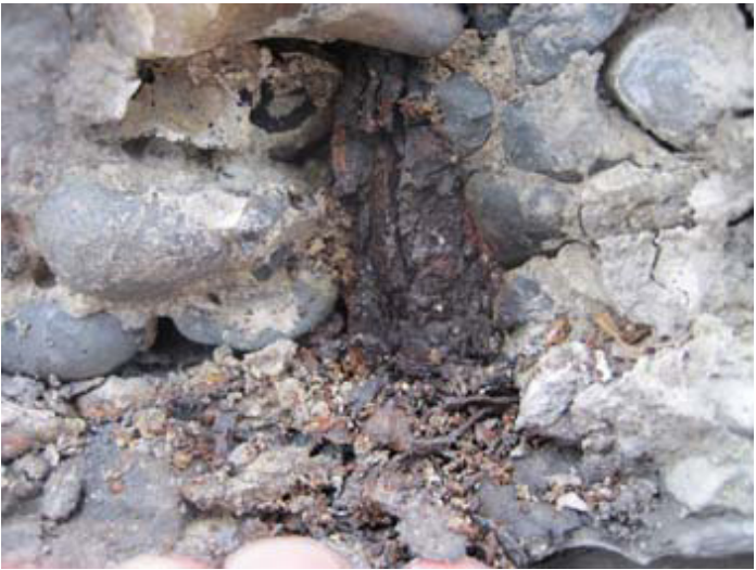
Spall and rusted reinforcing at exterior concrete wall
