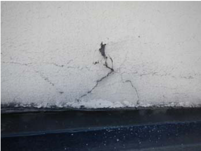
Cracking at exterior side of concrete wall
