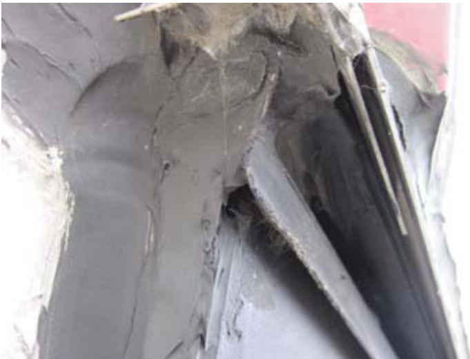
Multiple layers of sealant applications
