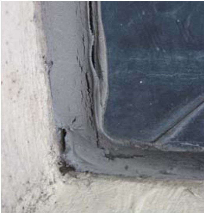
Failed sealant at punched window perimeter joint
