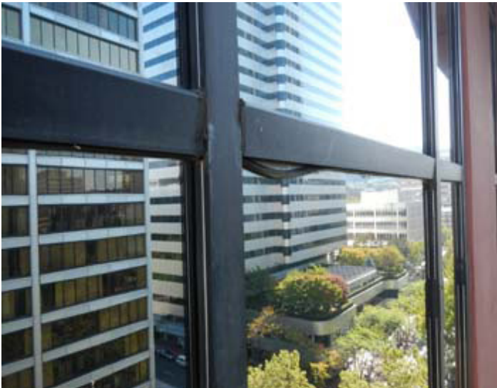
Failed gasket and displaced pressure plate/cap at curtainwall
