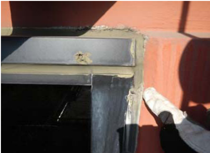
Sealant applied under head flashing
