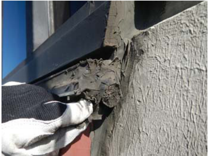
Multiple layers of sealant applications
