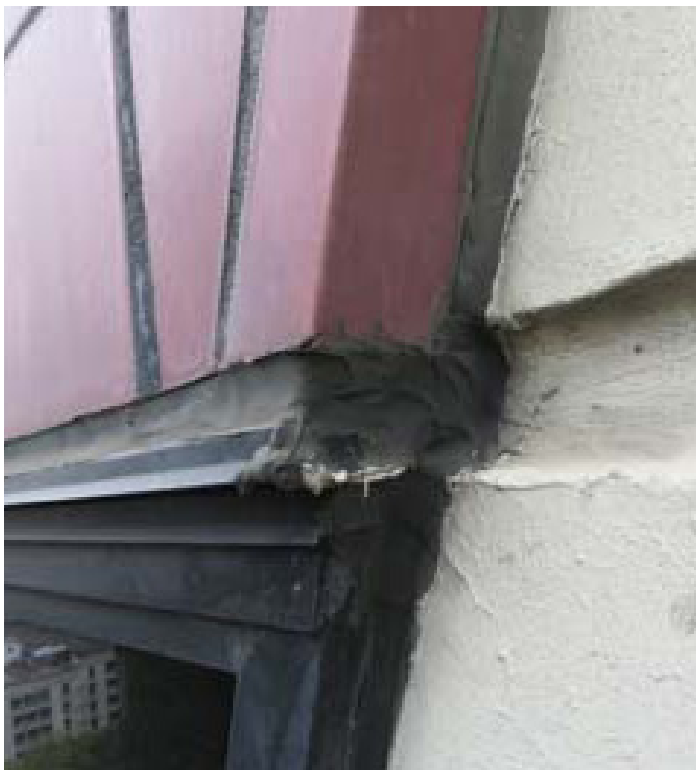
Ribbon window head below reveal
