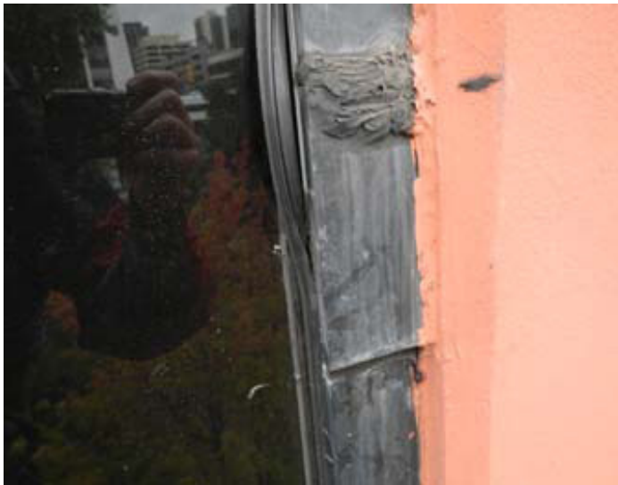
Failed movement splice connection at curtainwall jamb
