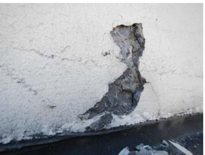
Spall at exterior side of concrete wall
