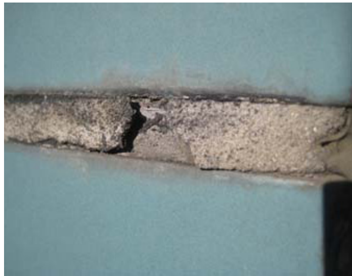
Failed grout in joint/efflorescence
