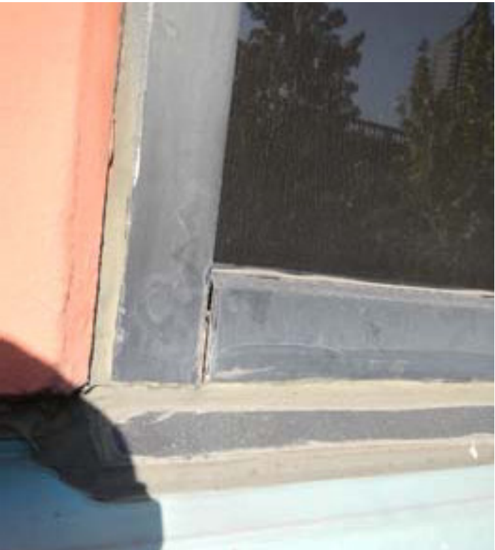
Sealant applied over curtainwall drainage outlet
