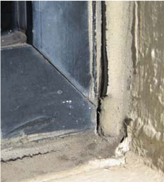
Adhesive and cohesive sealant failure
