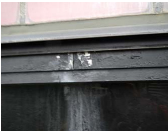
Failed metal finish at ribbon window head
