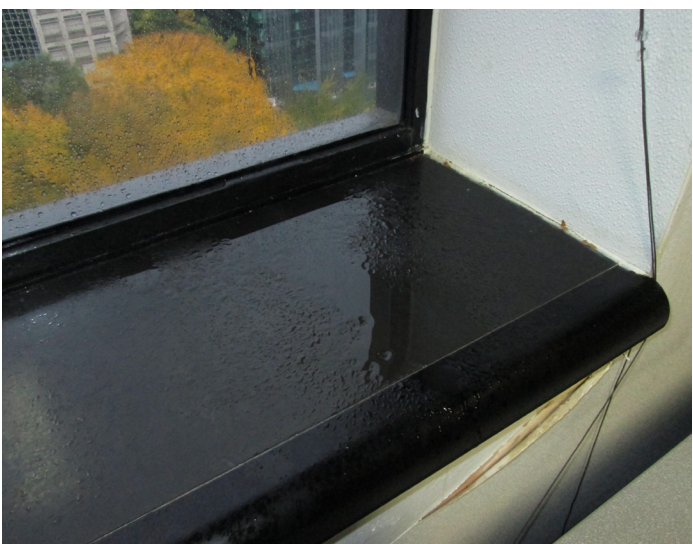
Water infiltration at 14th floor ribbon window
