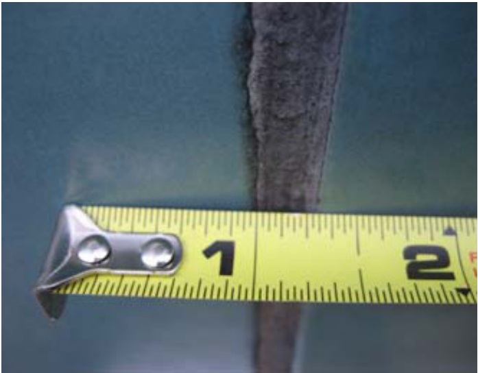
Irregular grout joint size
