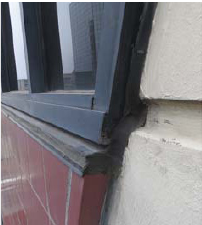
Ribbon window sill aligned with reveal
