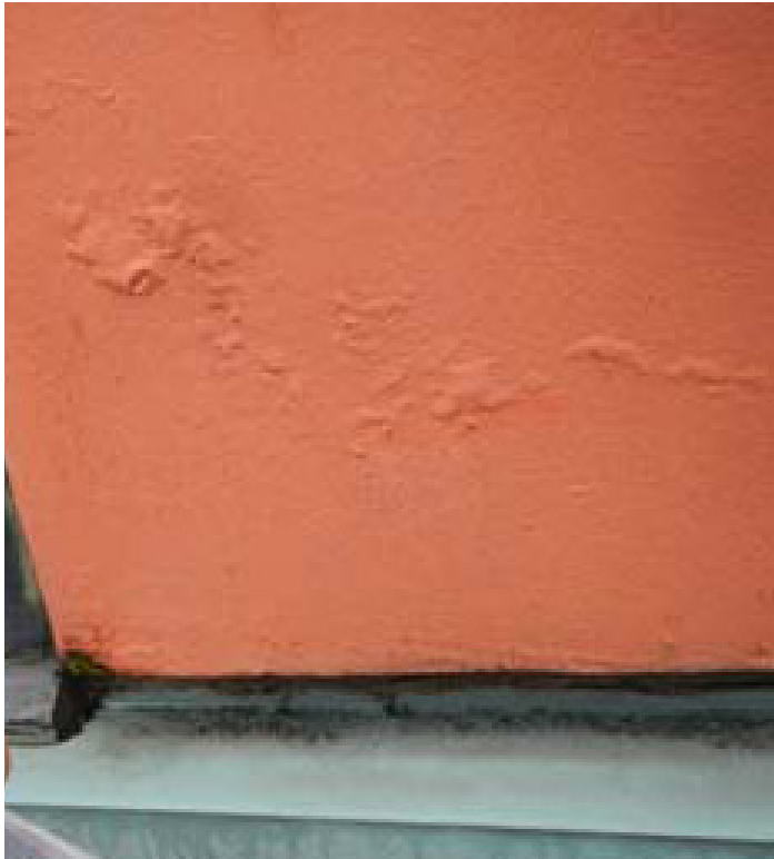
Bubbling at elastomeric paint
