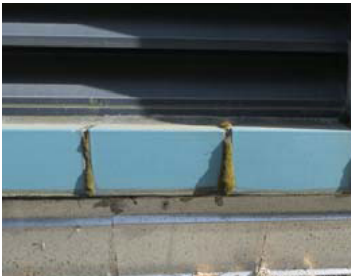
Biological growth at grout in joints
