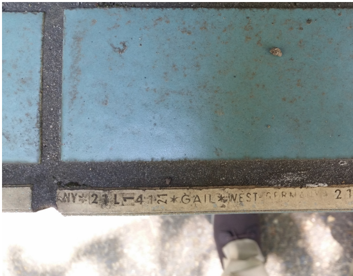
Field tiles modified for a corner condition
