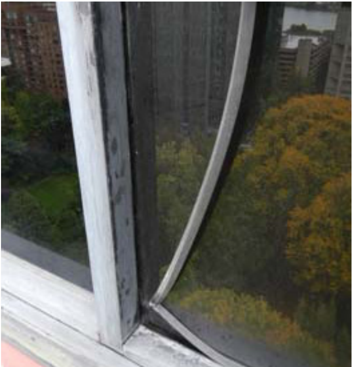
Failed gaskets and oxidized finish at ribbon window frames
