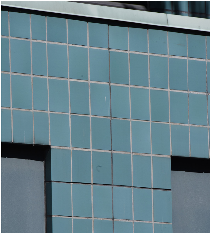
Tiles cut to different widths to maintain alignment
