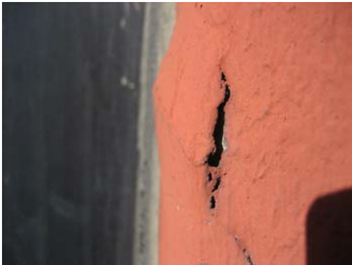
Failed elastomeric paint and loose concrete edge
