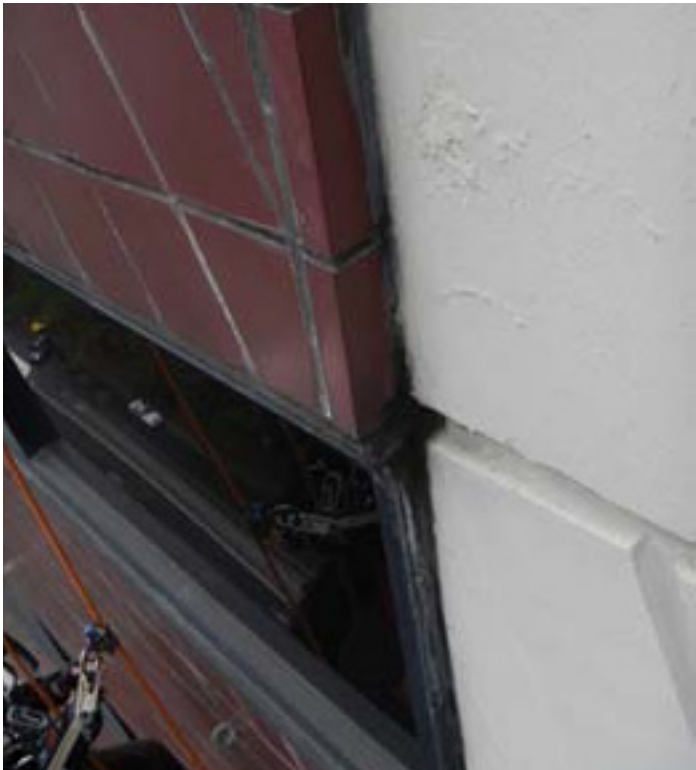
Weather tightness of transition dependent on sealant
