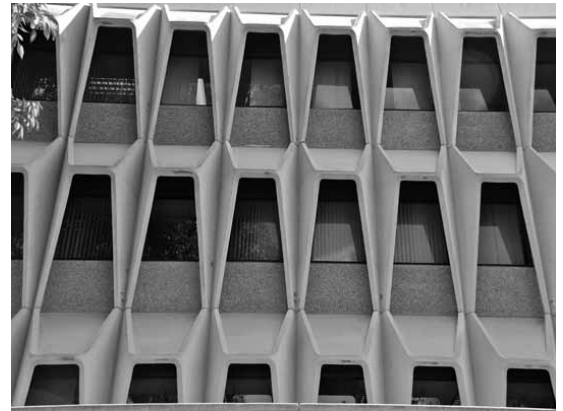
Detail of the shadows created by the precast sunshades. Steinhaus Hall, UC Irvine, Irvine, CA.
