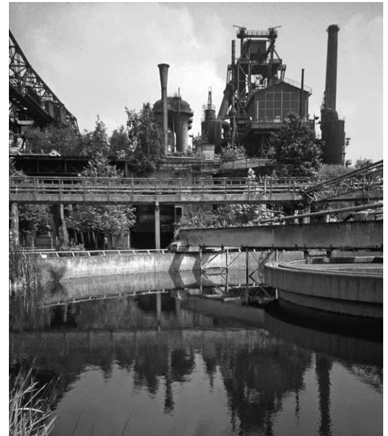
View of Latz's incorporation of thyssen Steelworks into the parks design. Landschaftspark, North-Duisburg, Germany. (photo: Franco Panzini)
