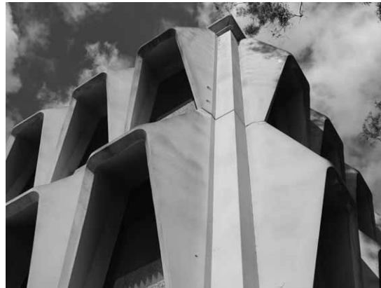
Detail of sculptural concrete sunshades on Steinhaus Hall, University of California at Irvine. Steinhaus Hall, UC Irvine, Irvine, CA. (photo: DOCOMOMO NOCA)
