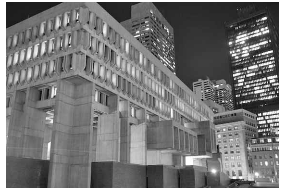
Detail view of the building's sculptural volume. Boston City Hall, Boston, MA. (photo: Chris Brazee)
