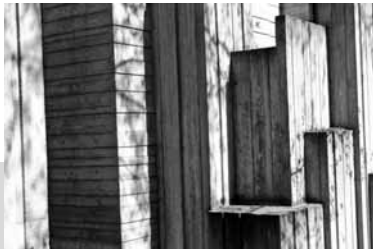
The shadows of the liriiodendron trees overhead play against the high relief of the board formed concrete. Freeway Park, Seattle, WA. (photo: Brice Maryman)
