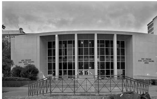
View of the building’s entrance now called the State Office Building Annex. LA Supreme Court Building at Duncan Plaza, New Orleans, LA. (photo: Neil Alexander)
