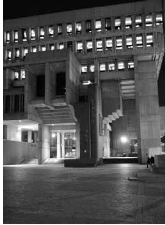
The building was constructed using mainly poured-in-place and precast Portland cement. Boston City Hall, Boston, MA. (photo: Chris Brazee)
