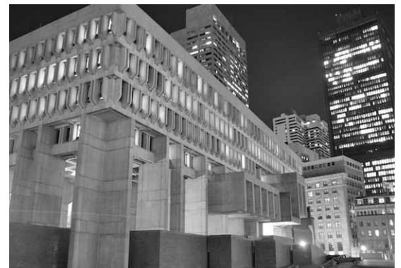
Detail view of the building's sculptural volume. Boston City Hall, Boston, MA. (photo: Chris Brazee)
