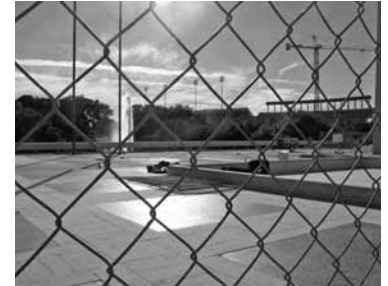
Detail of library plaza through construction. LBJ Library, Austin, TX. (photo: Catherine Gavin)
