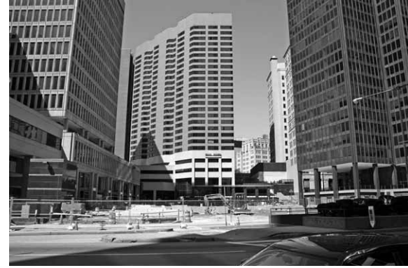
Center Plaza under construction, April 2007. Charles Center, Baltimore, MD (photo: Olivia Klose)
