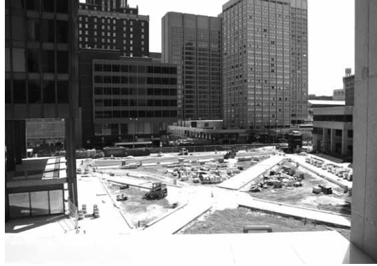
Center Plaza under construction, with Mies van der Rohe's One Charles Center on the right, April 2007. Charles Center, Baltimore, MD (photo: Olivia Klose)
