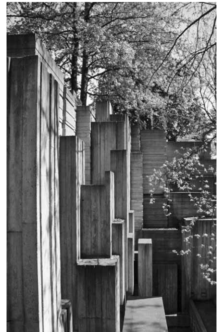
The current view into the canyon fountain shows the leaping concrete forms that became the hallmark of Freeway Park's hardscape vocabulary.
