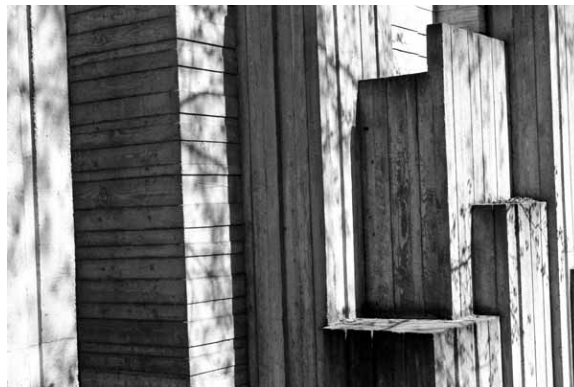
The shadows of the liriodendron trees overhead play against the high relief of the board formed concrete. Freeway Park, Seattle, WA.
