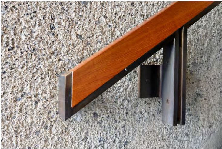
Staircase Detail Photo: John Arbuckle August, 2023
