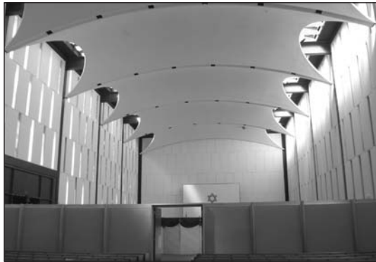
This view toward the rear of the sanctuary with its temporary partitions shows the shallow plaster vaults that help define each vertical bay.
