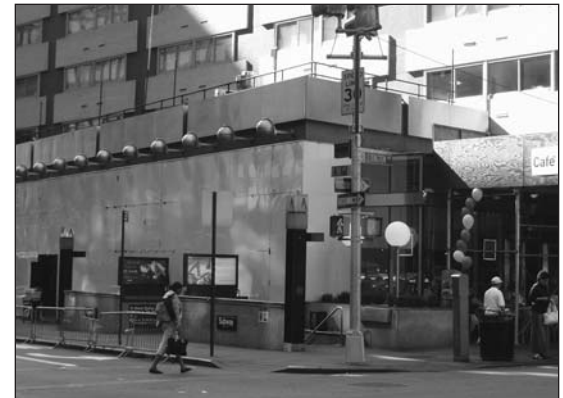
Summer 2005. White marble aggregate panels separated by narrow rules of dark green mosaic tile have been covered over with shiny white opaque glass squares. Sidewalk seating for the coffee shop now fills much of the open sidewalk space.
