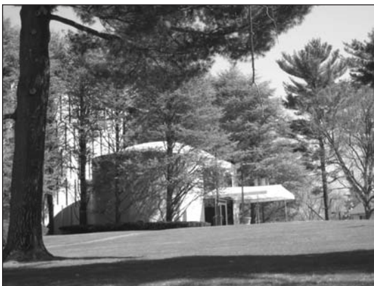
Kneses Tifereth Israel's rectilinear sanctuary is complemented by an elliptical entry building. Clad in white marble, both buildings are striking in their pastoral setting.
