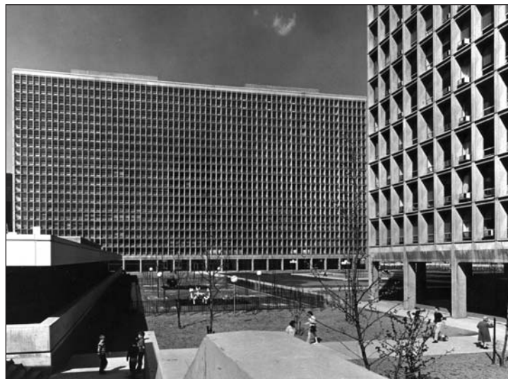
New and sparse in 1963. Today the two offset slabs combine with two newer perimeter buildings to create a more private courtyard that is lushly landscaped and shaded with 40-year-old trees—a true urban oasis.
