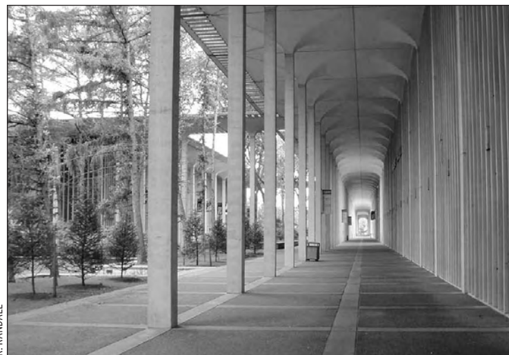
The campus required 270,000 cubic yards of concrete—much of which is finished in exposed aggregate. The variety of aggregates creates a subtle color variation between elements missing from monochrome views.
