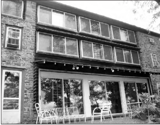
Rear elevation of the Raymond house—an 18th-century farmstead transformed c. 1940 by Antonin and Noémi Raymond.
