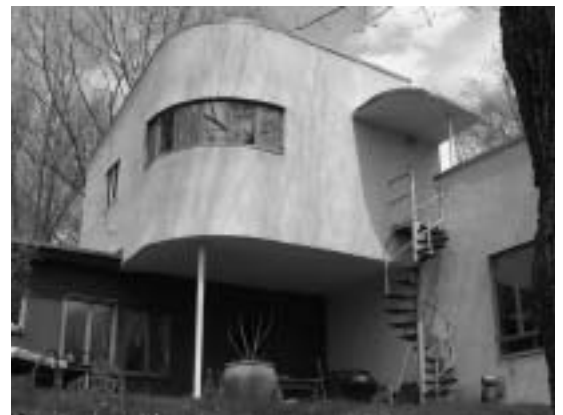
Detail, Field House, New Hartford, CT (photo: Dietrich Neumann)
